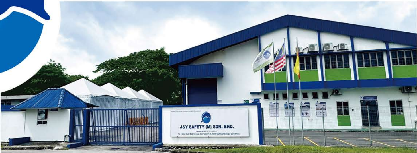
Oversea Plant J&Y SAFETY (M) SDN.BHD. (Malaysia)
